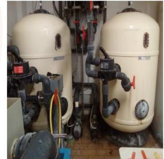
Mechanical, biological filters and UV lamp
